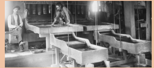
Gold extraction process using mercury to form an amalgam on copper plates.
