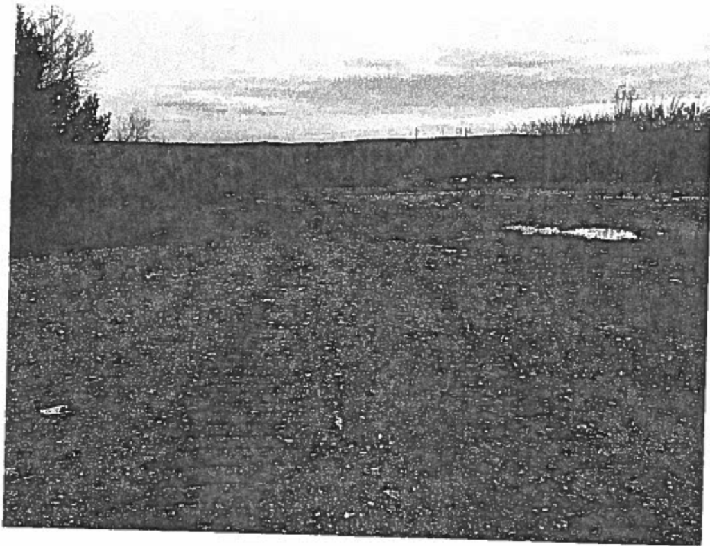
Photograph 1: View of the top of the slate fill embankment. December 5, 2017.
