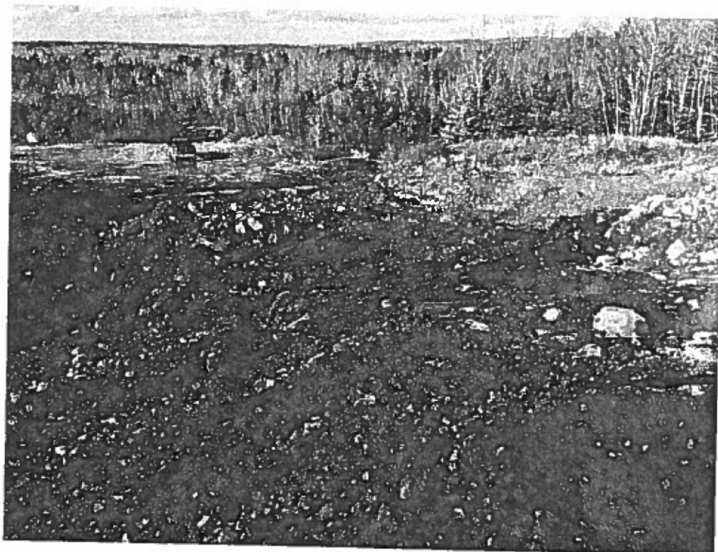
Photograph 12: View of the slate removal work. The slate was mostly removed except for the small stockpile in the background. December 14, 2017.
