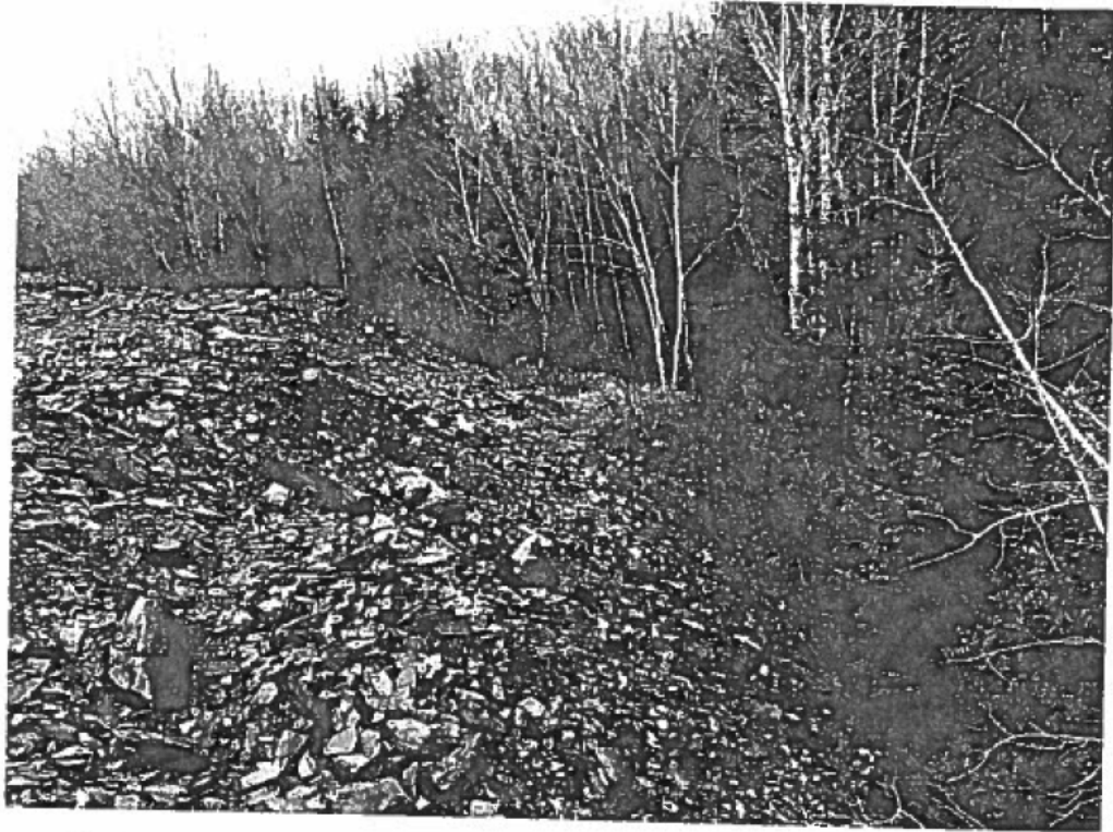
Photograph 3: View of the edge of the slate fill embankment (well-defined limit). December 5, 2017.
