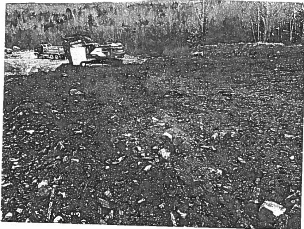
Photograph 8: View of the slate removal work well-underway. December 12, 2017.
