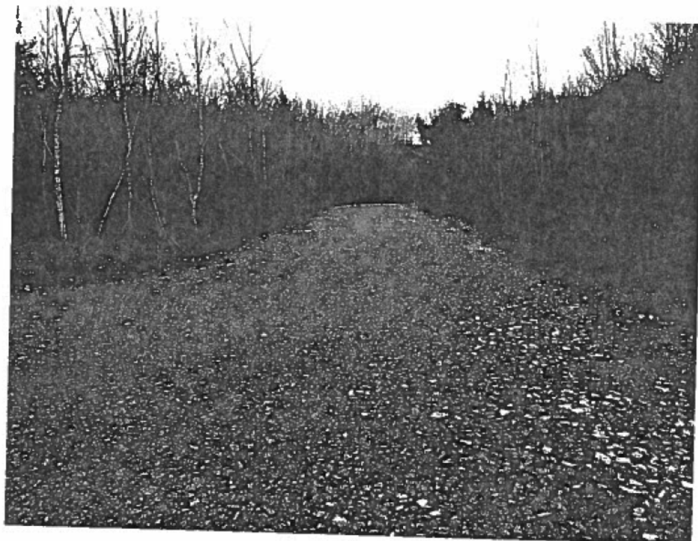
Photograph 6: View of the gravel access road from Waverley Road for truck access in preparation for the slate removal work. December 5, 2017.
