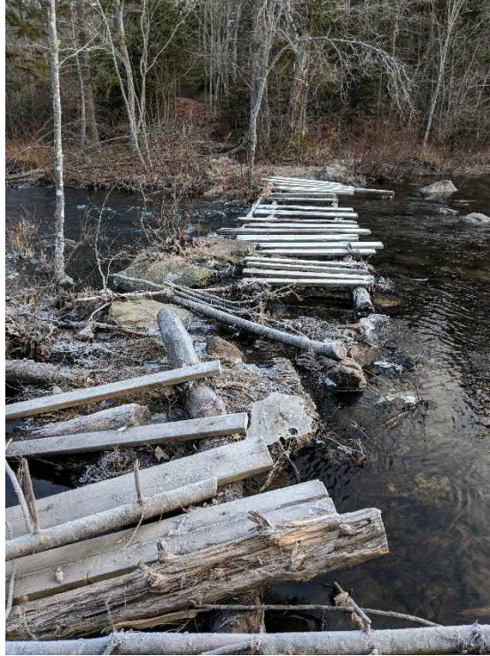
Photo 9. Small wooden bridge crossing Mitchell's Brook that is used for all-terrain vehicles (January 28, 2019).
