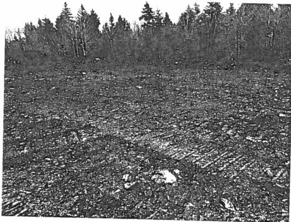
Photograph 10: View of the slate removal work. The slate is pushed to the edge of the area to allow for removal. December 12, 2017.
