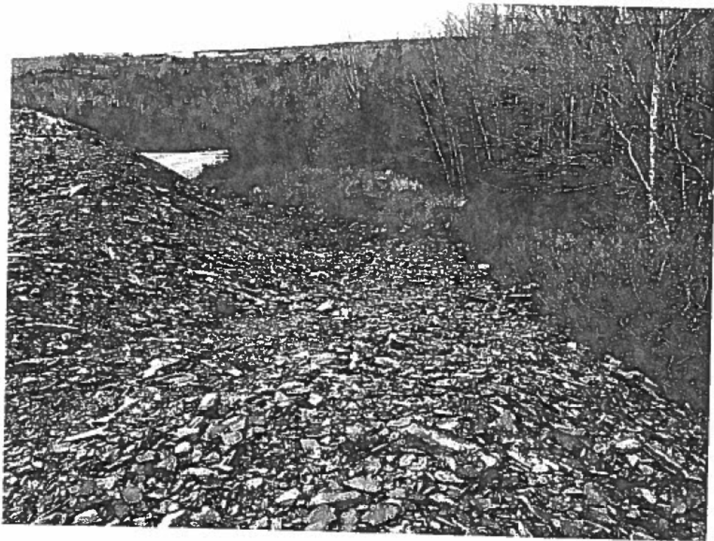
Photograph 4: View of the edge of the slate fill embankment (well-defined limit). December 5, 2017.
