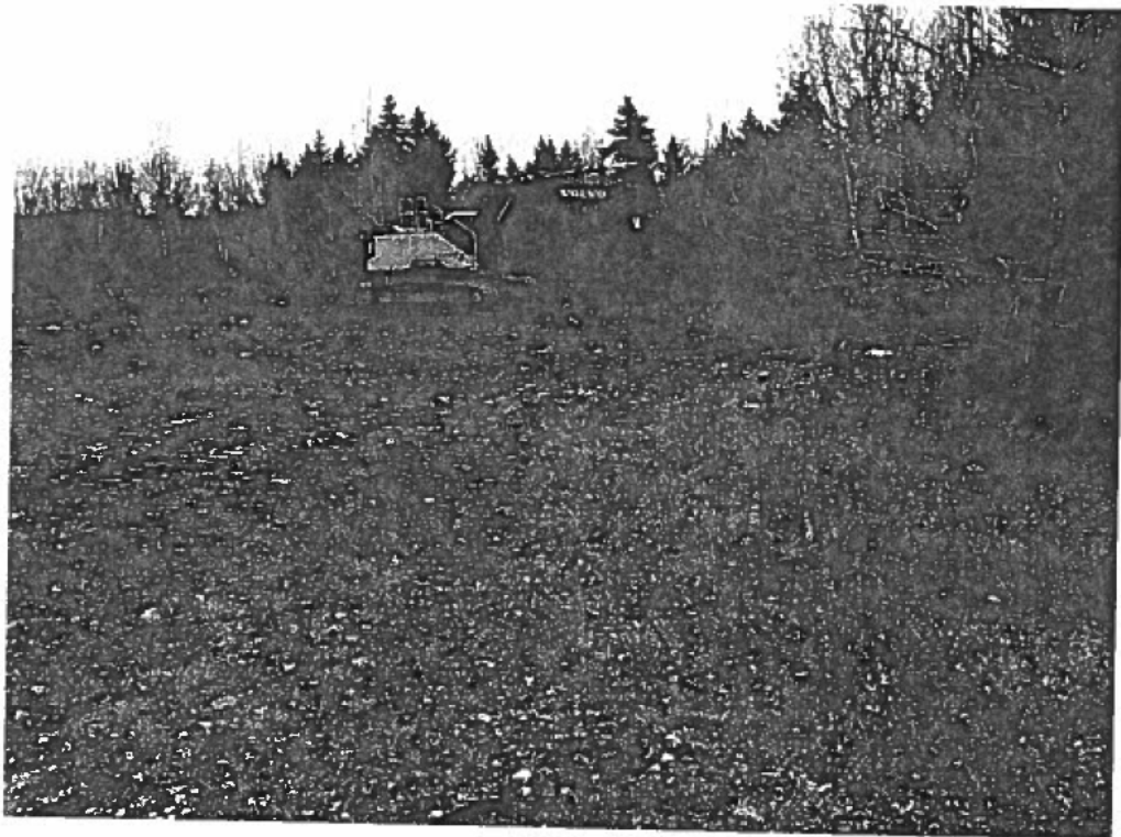
Photograph 11: View of the second excavator moving the slate at the edge of the stockpile/embankment area. December 12, 2017.
