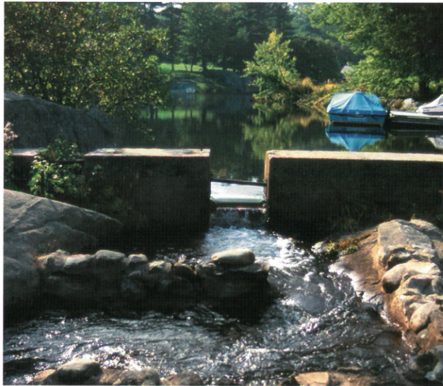
This alewife fishway on the Damariscotta River allows tens of thousands of alewife to make their annual spawning migration into Damariscotta Lake. Removal of this fishway would block the alewife migration, and eventually extirpate alewife floaters from the lake. ETHAN NEDEAU
